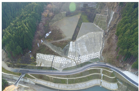
貯水池上流左岸法面对策
