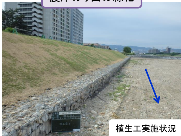
護岸のり面の緑化
